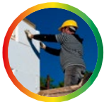
External wall insulation
